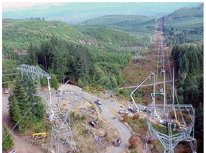
An overhead view of SnoKing Tap taken from a helicopter.
