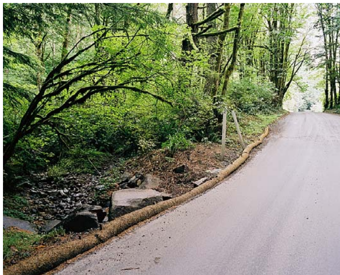
Netted bags filled with cedar chips line the roads inside the Cedar River Watershed to protect pollutants from entering land and waterways. The cedar chip bag has proven to be a very effective low technology model.
